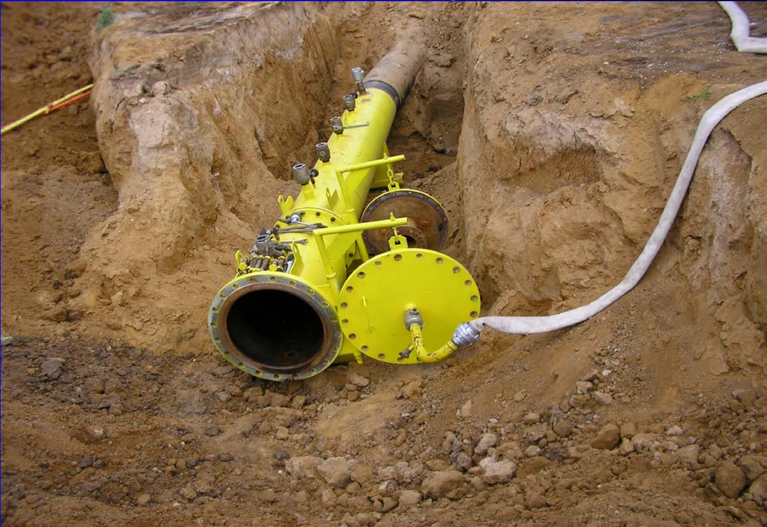
Several bi-di pigs was put into the temporary pig trap. The spaces between the individual pigs were stepwise filled by the Petrosol surfactant in different concentration.
